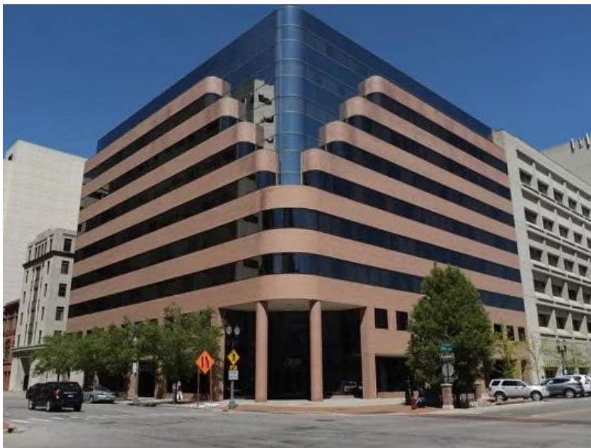
Victor Office Center, a Gentilozzi property at 201 N. Washington Sq. Monday, May 15, 2017. (Photo: Robert Killips | Lansing State Journal)
